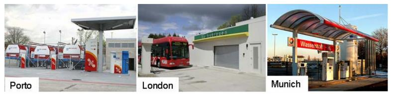
Filling stations have been built in 10 cities in Europe to support fuel cell buses in the EC CUTE<sup>1</sup> project. These stations are relatively large, able to refill at least 3 buses per day.
